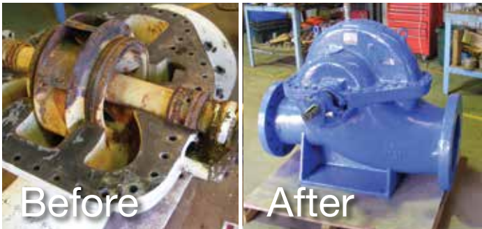
Overhaul of split case pump
